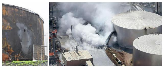
Figure 4 — Enormous hole several feet in diameter in an asphalt storage tank resulting from the April 26, 2018 Husky Superior Refinery Explosion in Superior, Wisconsin.
